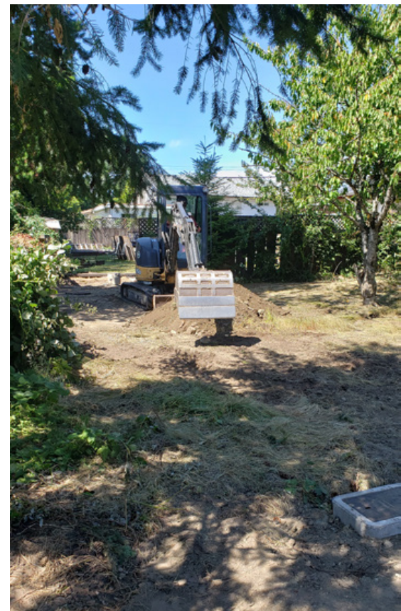
All work was done within the backyard easements
