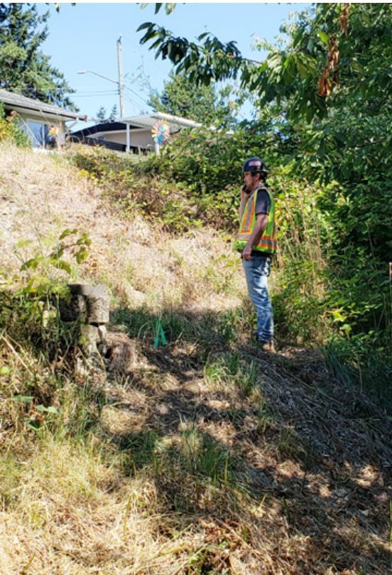
Challenges included steepness of the work areas
